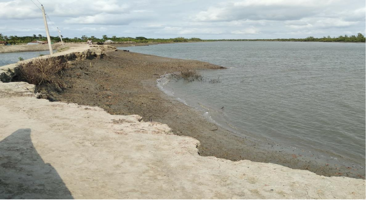
Climatic variabilities leading to disasters, including chronic river bank erosions
