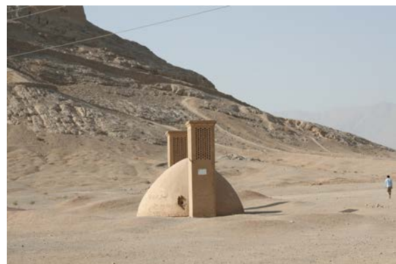
Photo 1. Drinking water tank (The water comes through the underwater canal) (Photo: Vafadarimehrizi Kazem)
